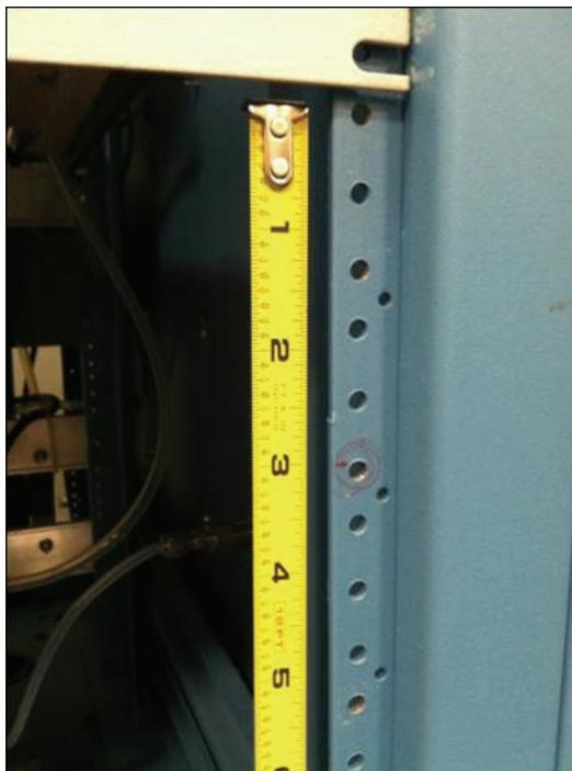
**Figure 2-2.** Slide Rail Mounting Holes
