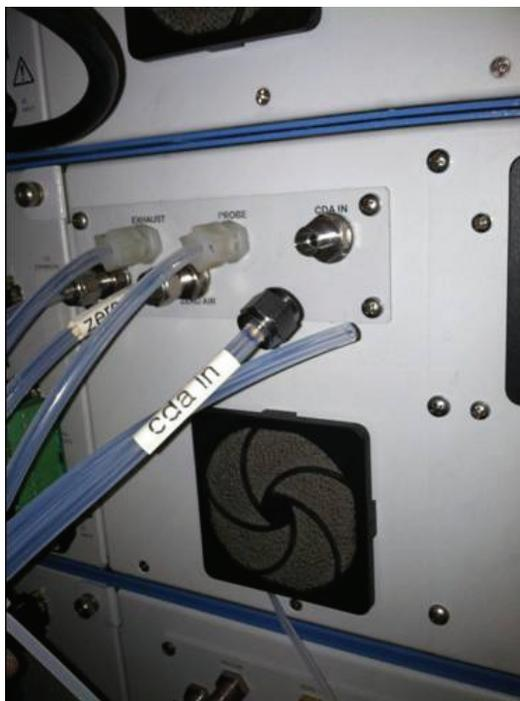
**Figure 2–4.** 81*i* CDA Line Removed
